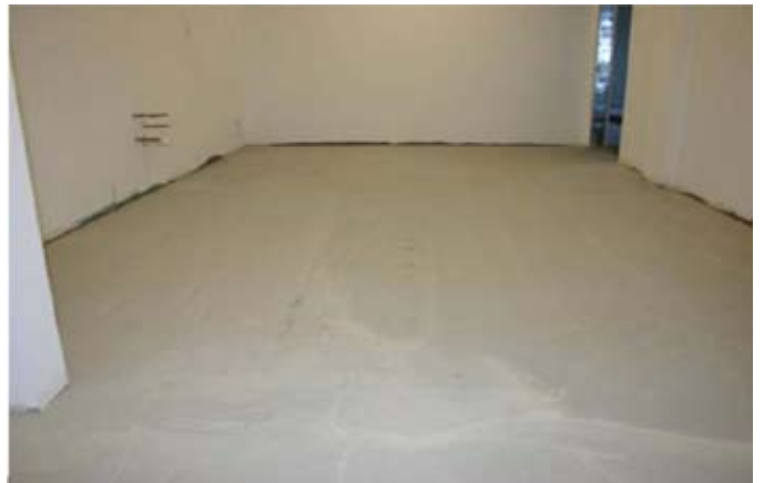
Element covered by floor leveler
