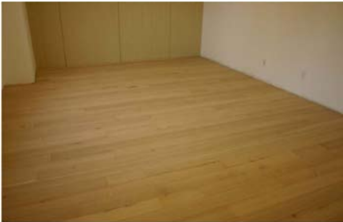
Work room - finished floor is floating wood boards
