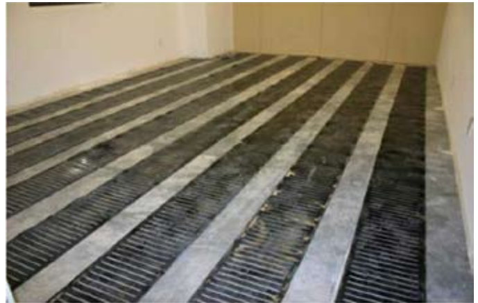
Elements on insulated concrete covered by a sound barrier
