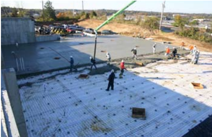
Heating Elements Over Insulation and Under 6" Slab
