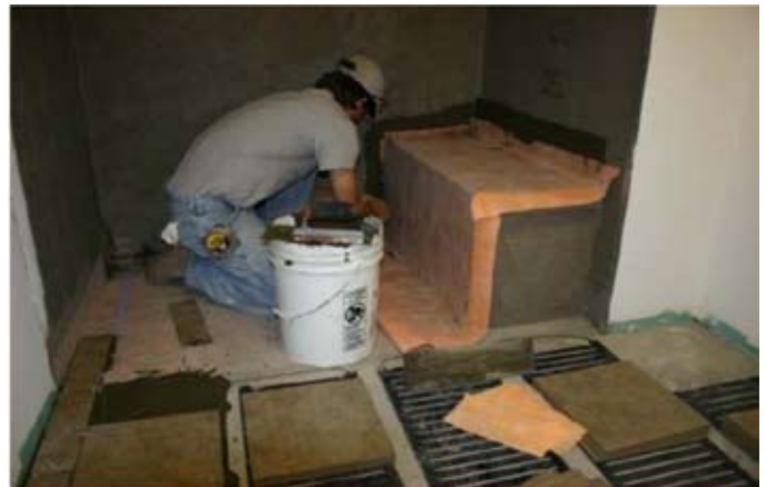
Heating on the floor and the bench
