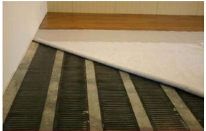
Elements on concrete, under sound barrier and bamboo
